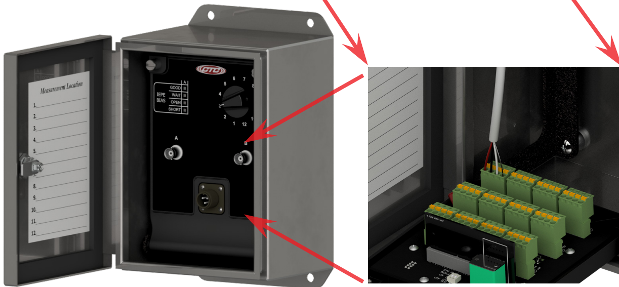
Figure 10. Field Wiring for 3-Conductor Sensor Inputs
