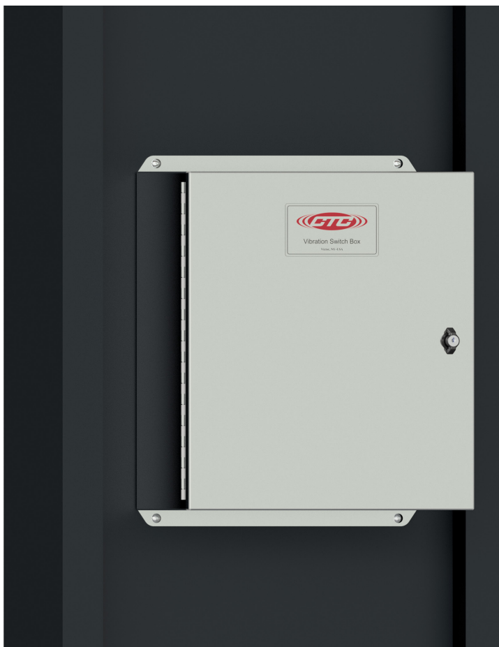
Figure 5. Switch Box (MX403) Earth Ground
